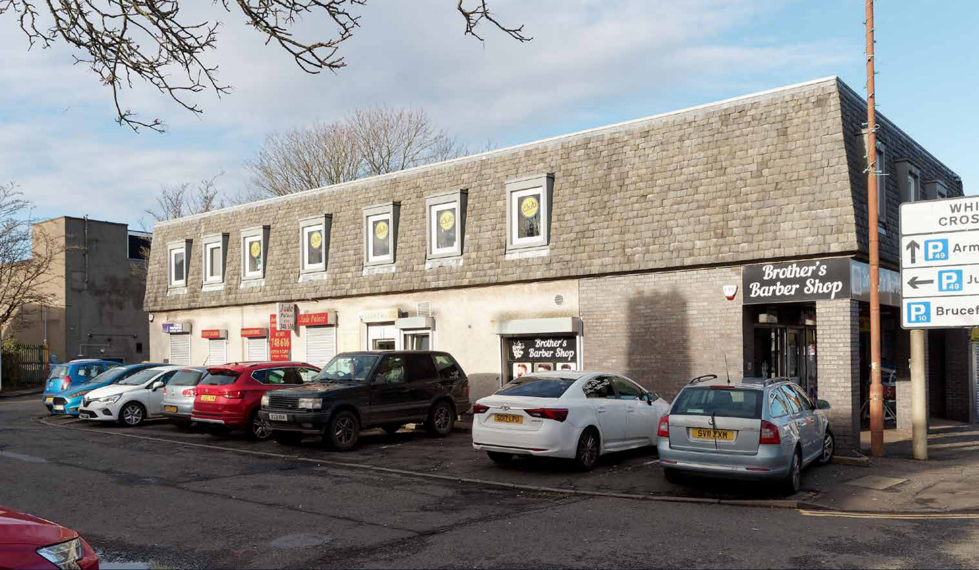
Barras House, 6 Manse Road, Whitburn, West Lothian, EH47 OQA
