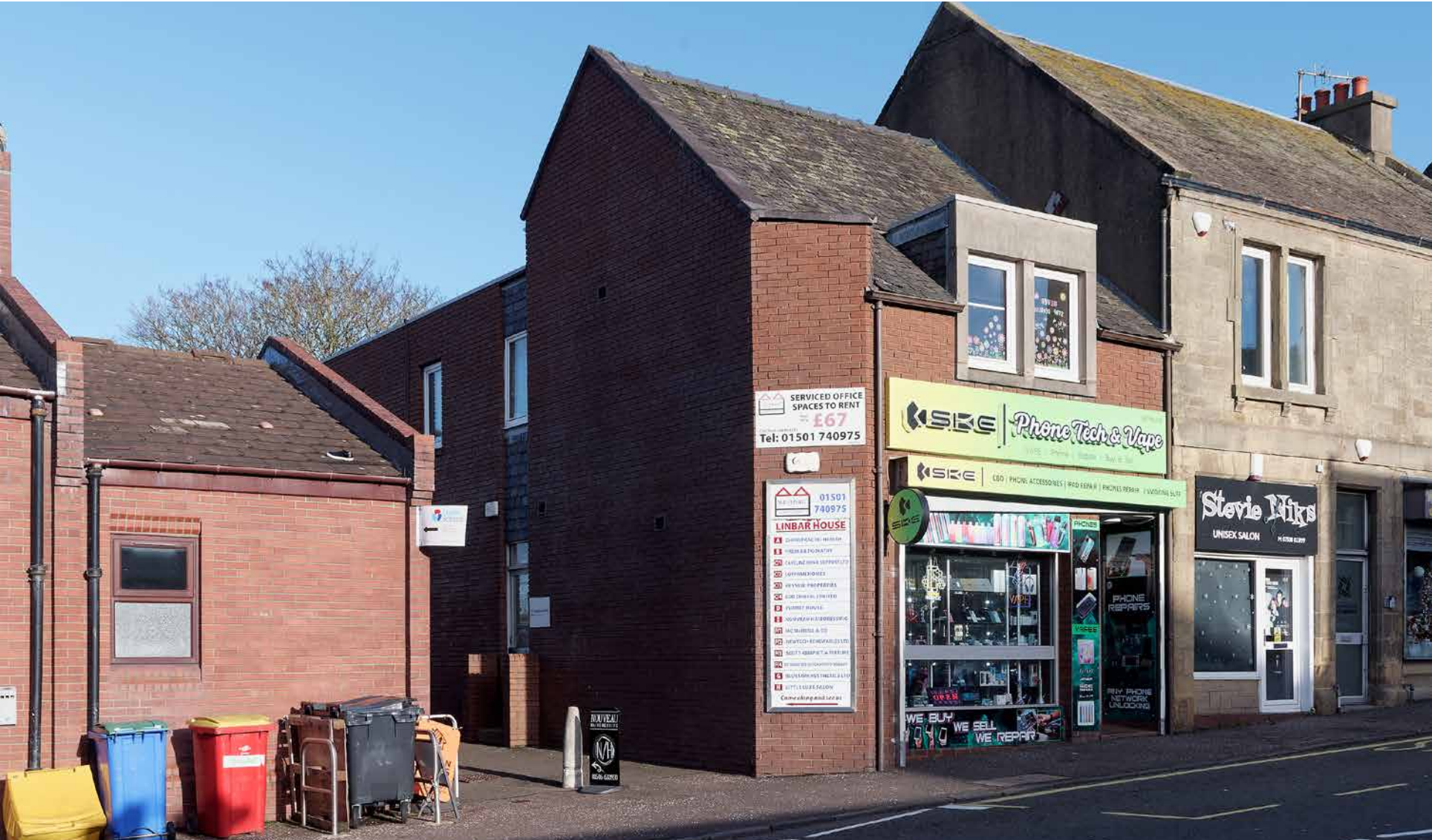
Linbar House, 48 North Bridge Street, Bathgate, West Lothian, EH48 4PP
